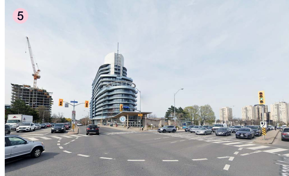
Sheppard Avenue East and Bayview Avenue Intersection, Looking Northeast
